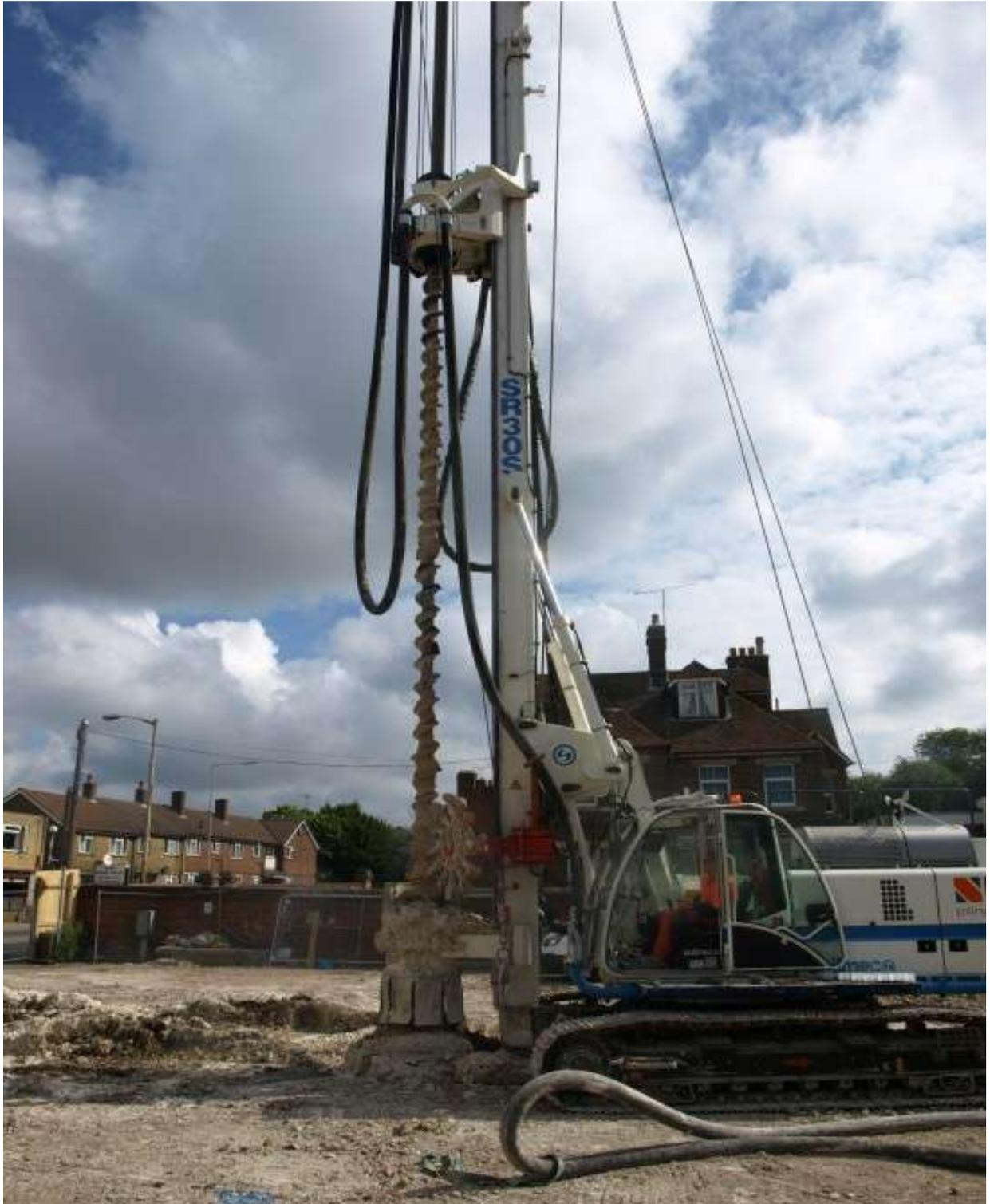
*Plate 13: Showing rig SR303 drilling pile no.43. Looking North.*
